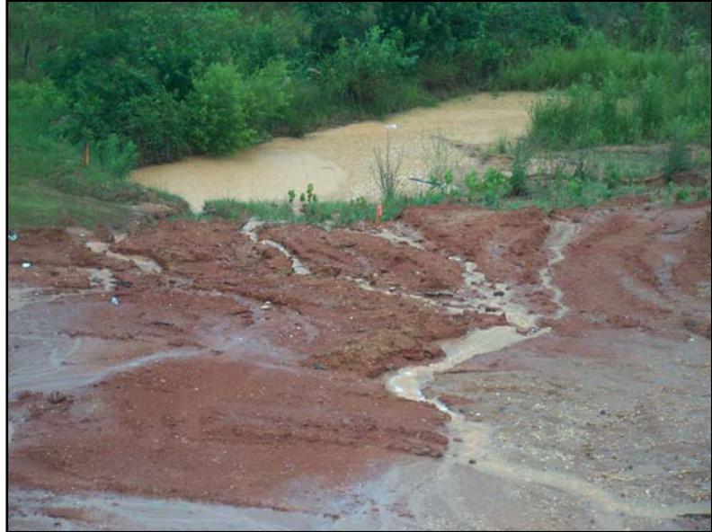
Soil erosion from construction site carrying pollutants into a stream
