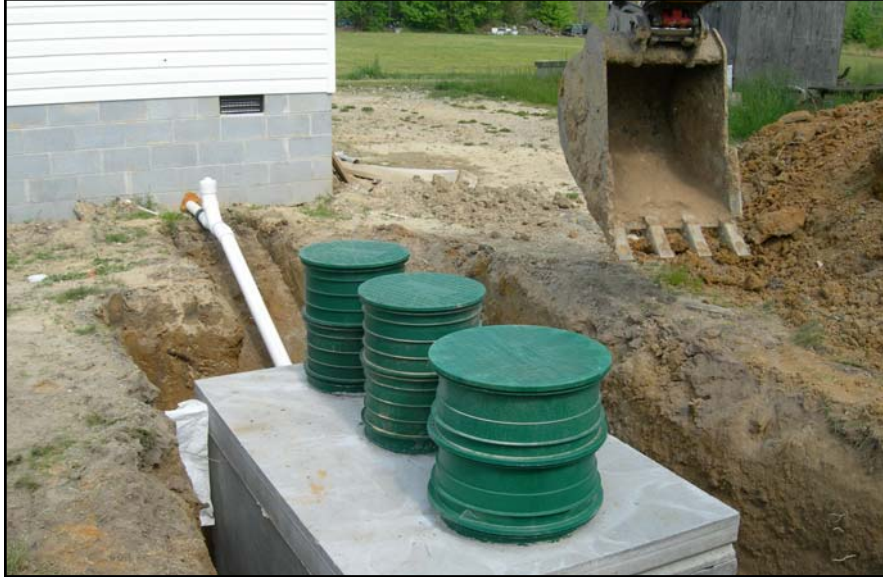
Replacement of a septic system in association with Dawn Project
