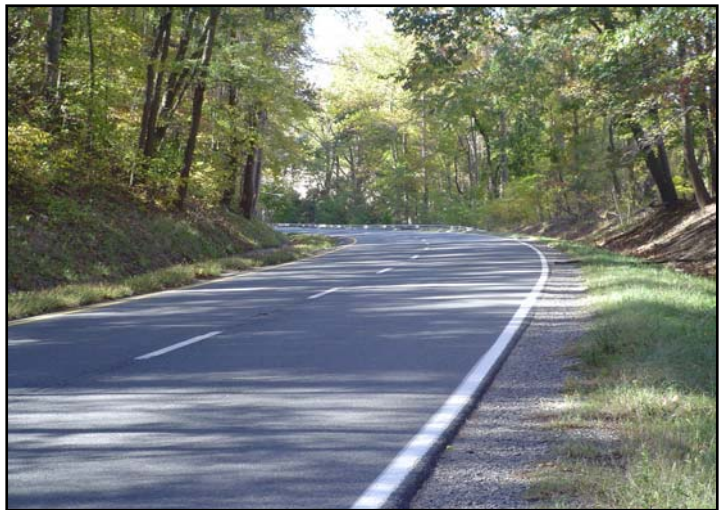
Tidewater Trail looking westbound near Camden
