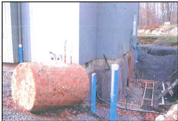
Underground Storage Tank after extraction
